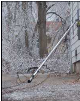
Damaged Weatherhead
